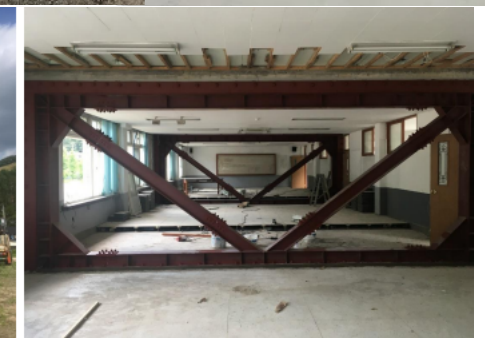
The reinforcement
