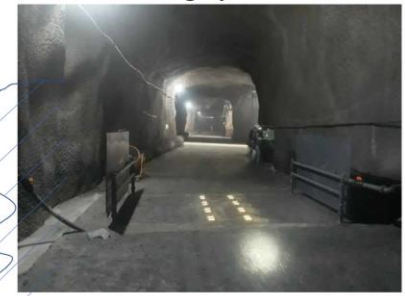
Car washing system (-35m)
